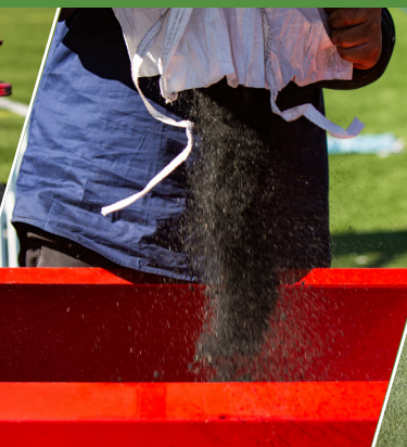
Infill Top Up in progress
